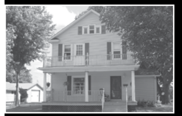
309 East 3rd Street
